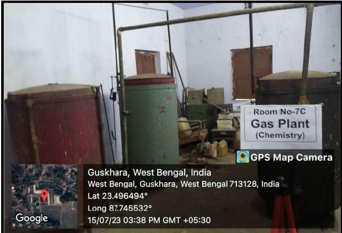
Figure-81: Gas Plant (Chemistry)
