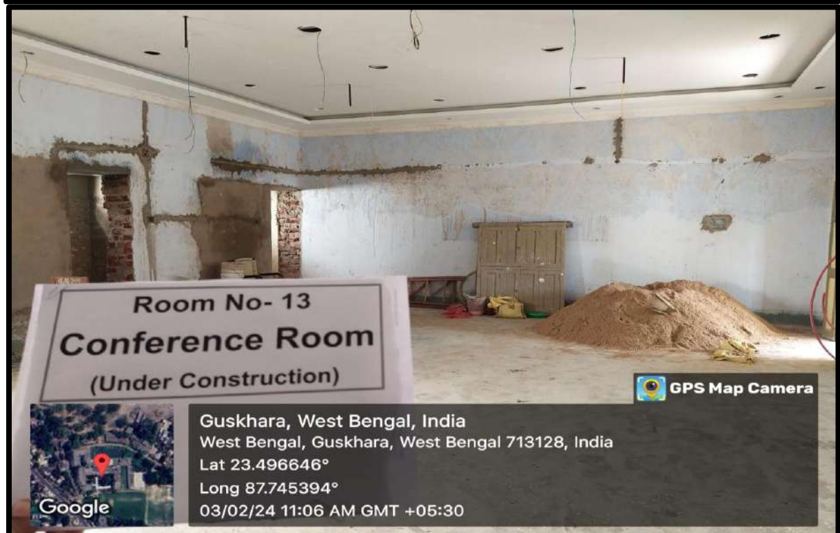
Figure-38: Conference Room (Under Construction)
